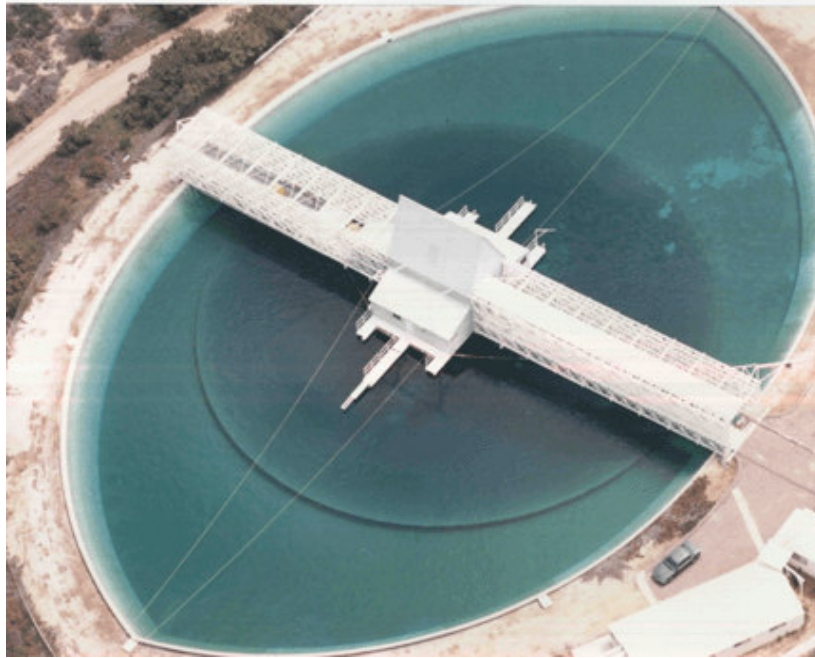
Figure 1: Aerial photo of facility. The water clarity shown is typical. The bridge structure has no piers or supports in the pond and does not obstruct the water
