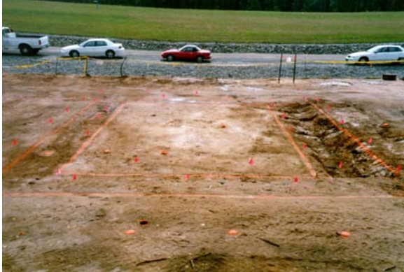
Figure 15 Zone of injection of the barrier
