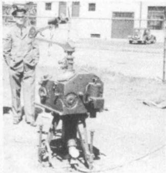
3. Comparator and searchlight control are in one unit. Comparator corrects data from locator and control unit moves searchlight accordingly. Light is operated by remote control to protect personnel, since it will be subjected to enemy strafing.
