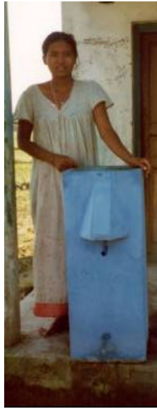
Fig 2. An existing Biosand filter in Nepal
