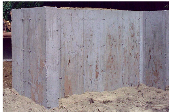
Fig. 12. The 10 cm thick solid concrete test wall.
